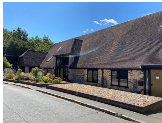
Fig 33: Domestic character of barn and setting
