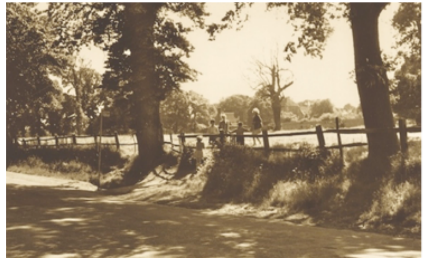
Fig 3: Historic (undated) photograph of view from Kingston Lane south towards St Julian's Church
