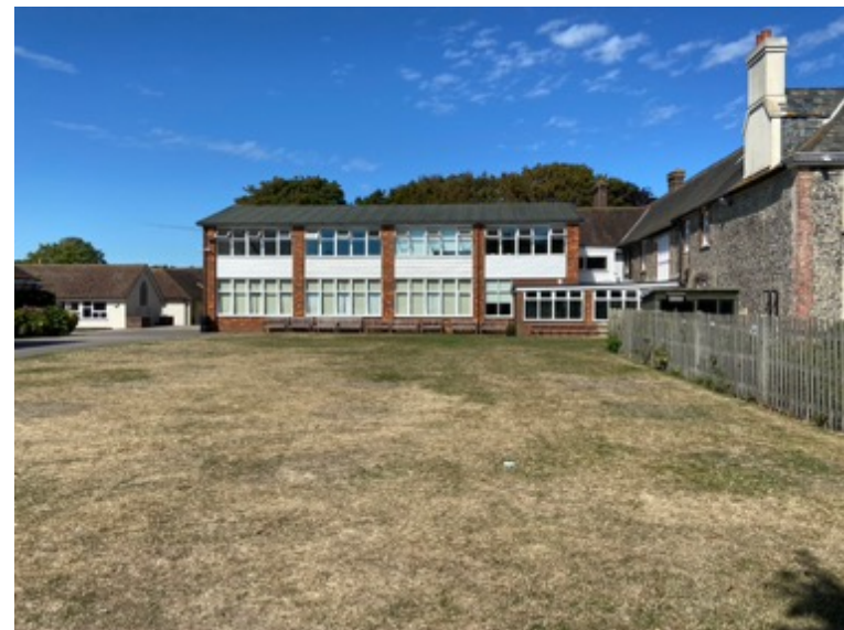
Fig 31: Disproportionate additions and inappropriate alterations to historic buildings
