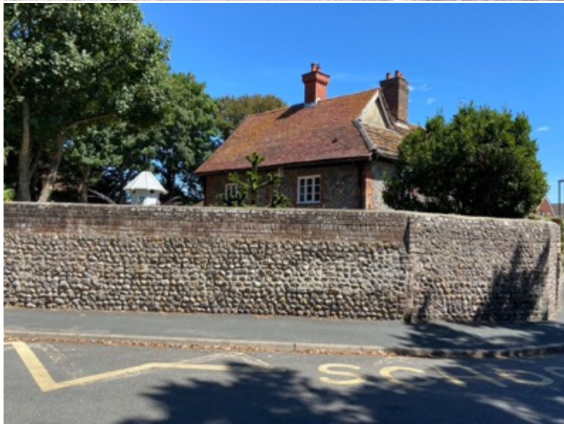
Fig 13: Flint walls, flint buildings with brick dressings and tiled roofs
