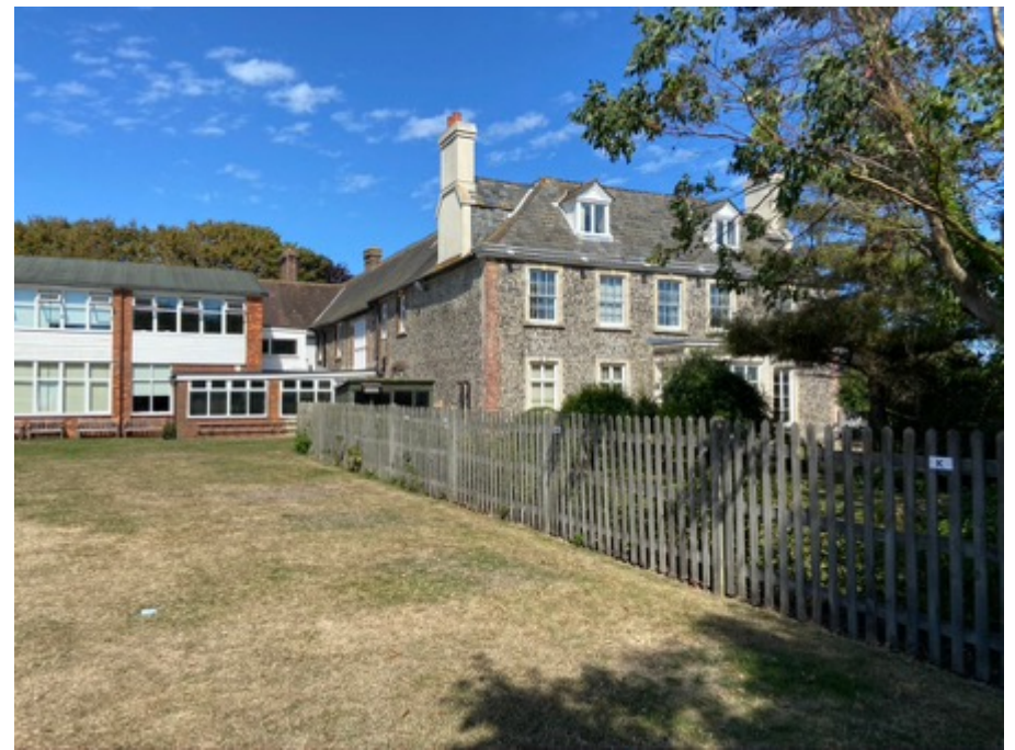
Fig 14: Knapped and coursed flint, slate roof
